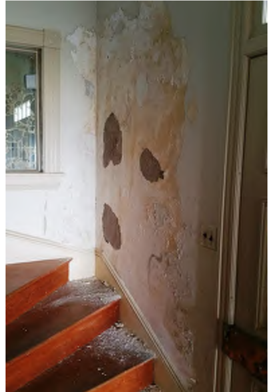
Plaster damage from moisture issues
