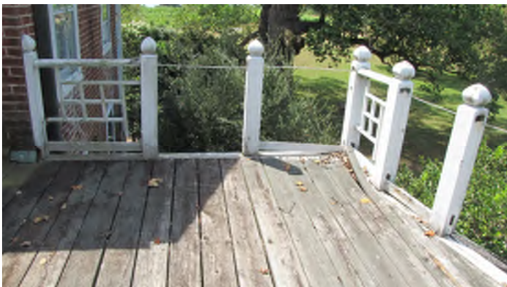
Deteriorated second floor deck and railing
