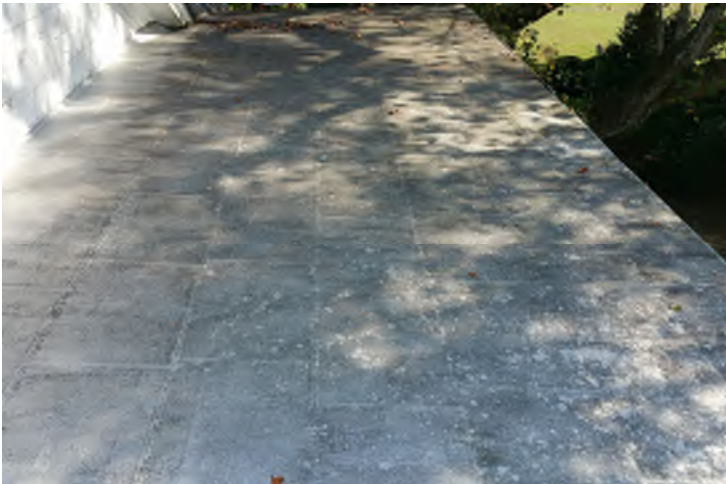
Flat seam metal roof at porch
