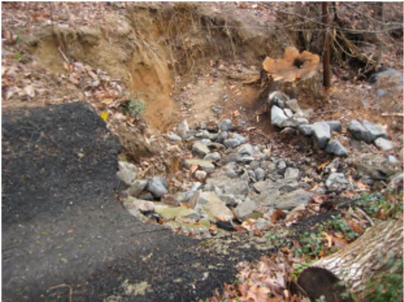
Broken, Eroding Paved Ditches
