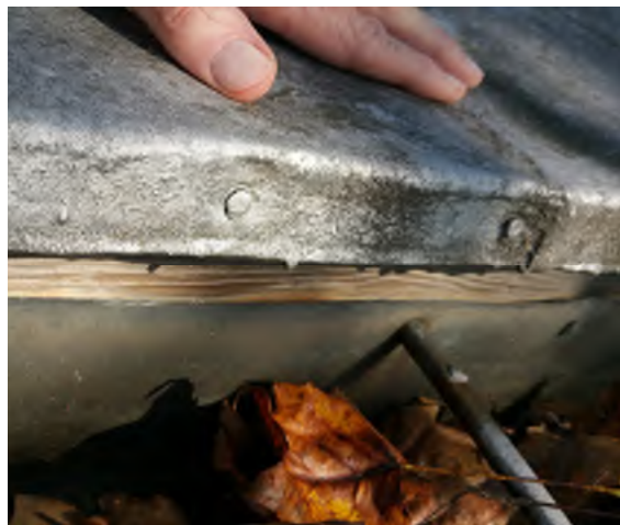
Rework detail at porch roof edge/gutter
