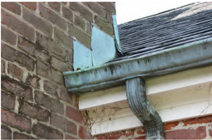
Gutter at garage and main house overflowing
