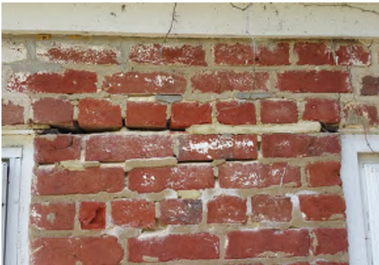
Servant Quarters improper mortar repairs & corroded lintel
