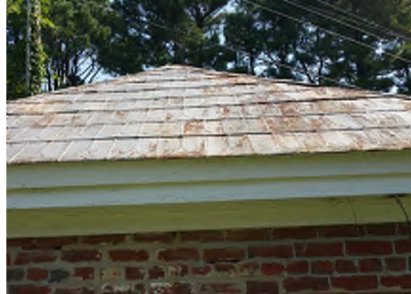
Smokehouse roof deterioration
