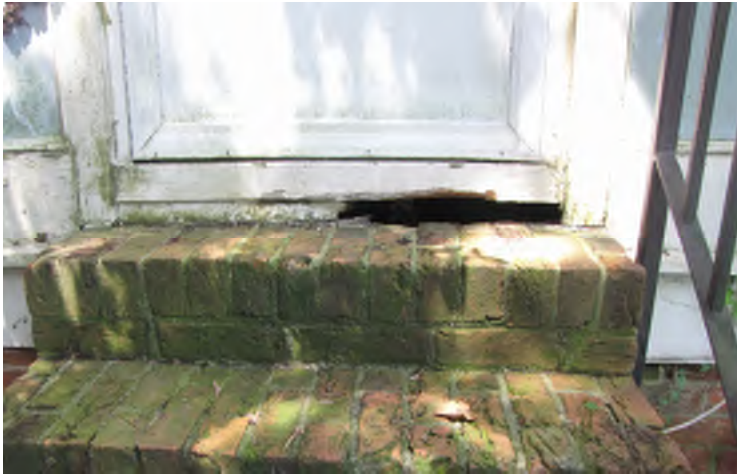
Rot at south entry to porch
