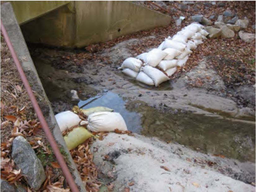
Excessive Erosion from Uncontrolled Runoff
