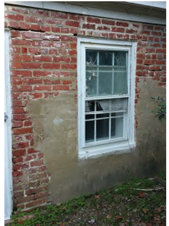
Brick Issues at Servant Quarters
