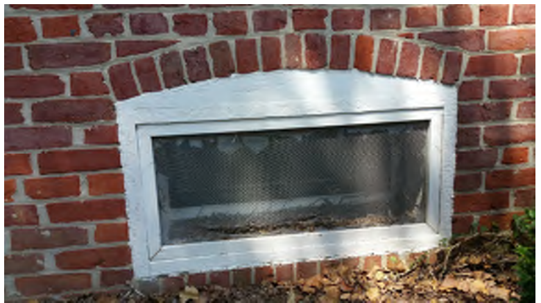
Typical Basement window with screen
