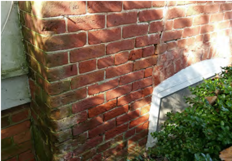
S corner of house by porch steps
