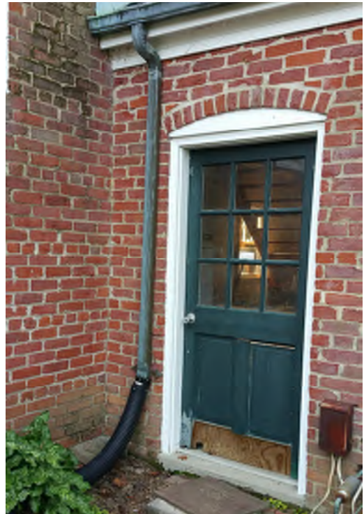
Deteriorated garage door
