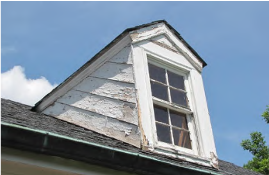
Wood damage/rot on Amblers House
