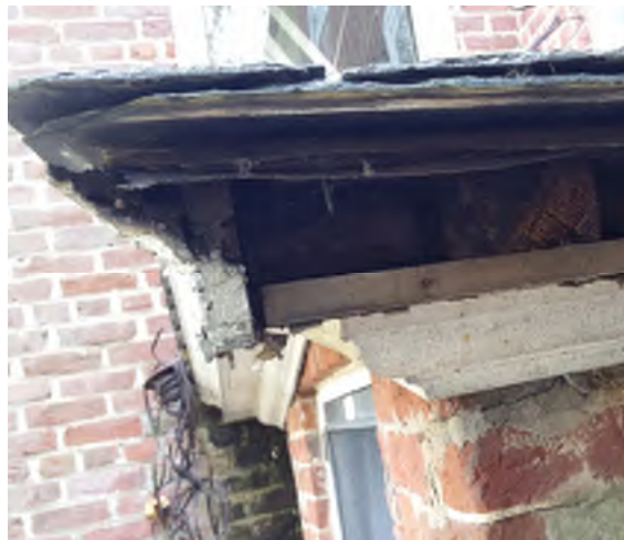
Basement bulkhead trim rot
