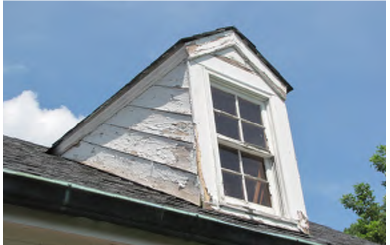
Wood damage at garage dormer
