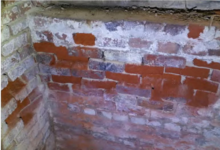
“Rising Damp” deterioration in basement
