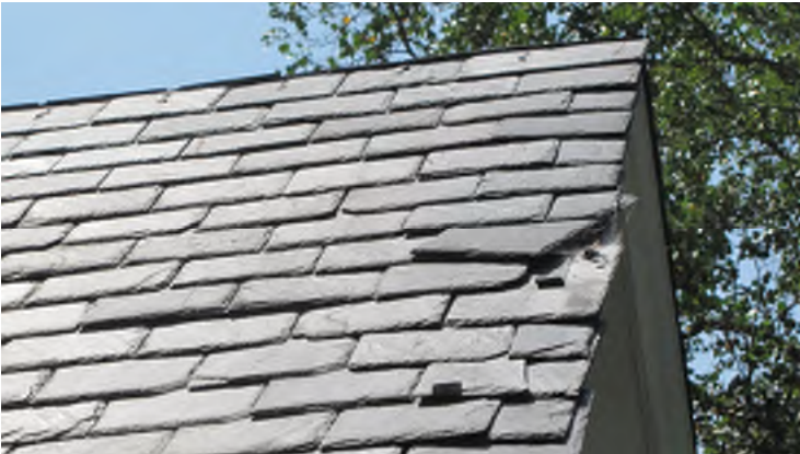
Damaged slate
