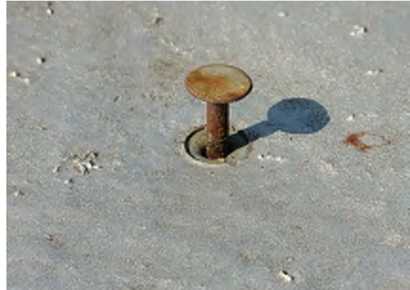
Nail in porch roof repair area
