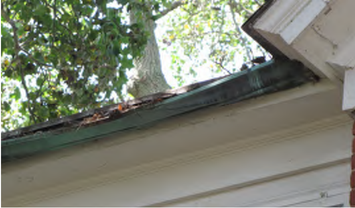
Damaged gutter at porch
