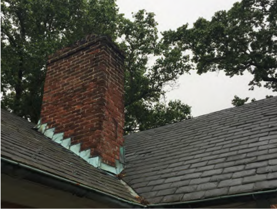
Roof and chimney of Amblers House
