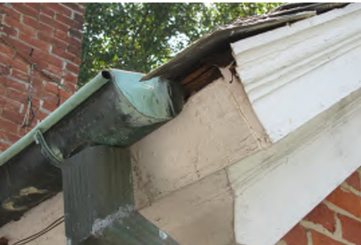
Trim rot above 2nd floor deck
