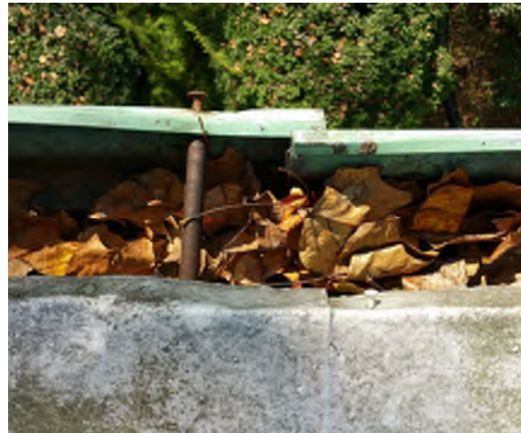
Gutters at porch roof needing repair
