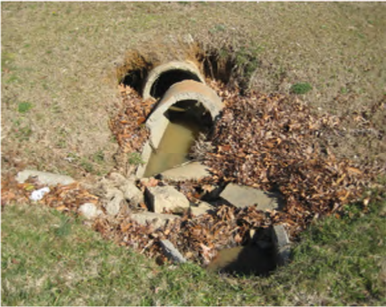
Aging, Failing Storm Drains
