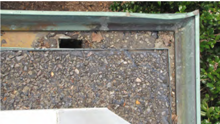
Built-up roof under second floor deck
