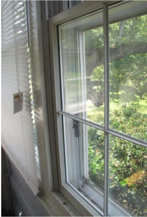
Newer windows at porch
