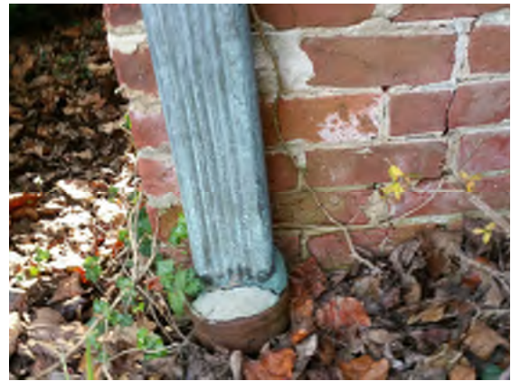
Downspout into underground storm pipe
