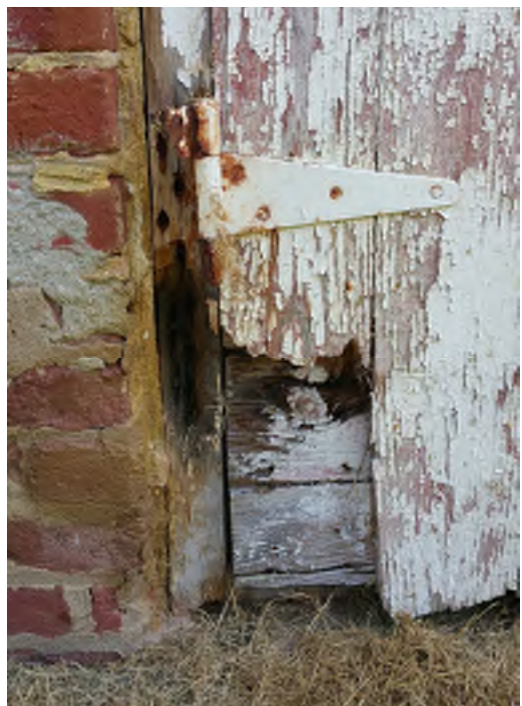
Smokehouse door deterioration
