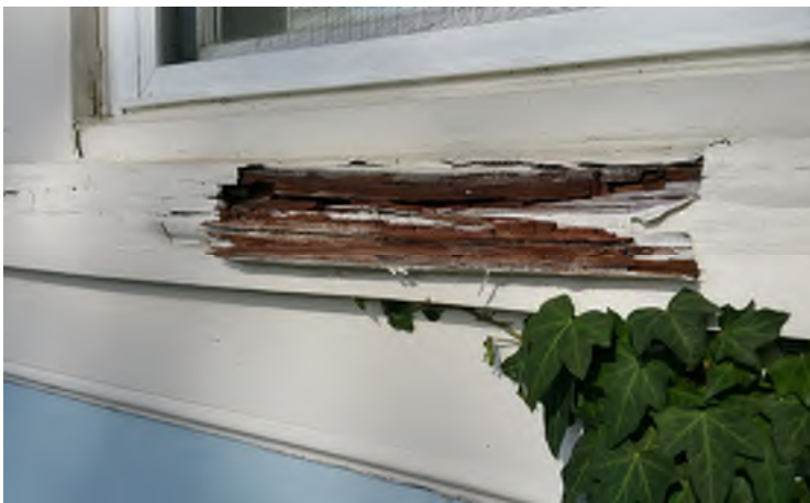
Rot at porch window sill
