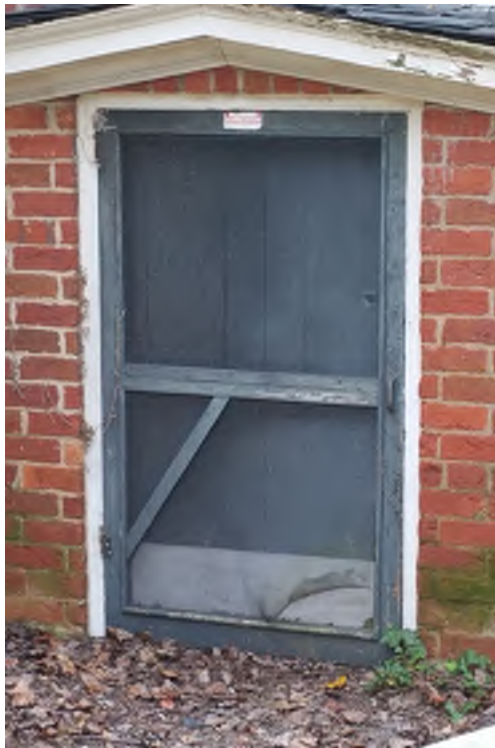
Screen Door deterioration at bulkhead
